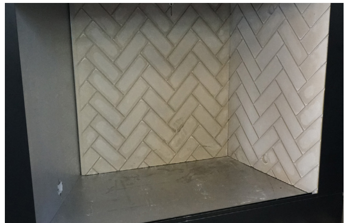
Install Right Side Refractory Brick Liner Figure 49
