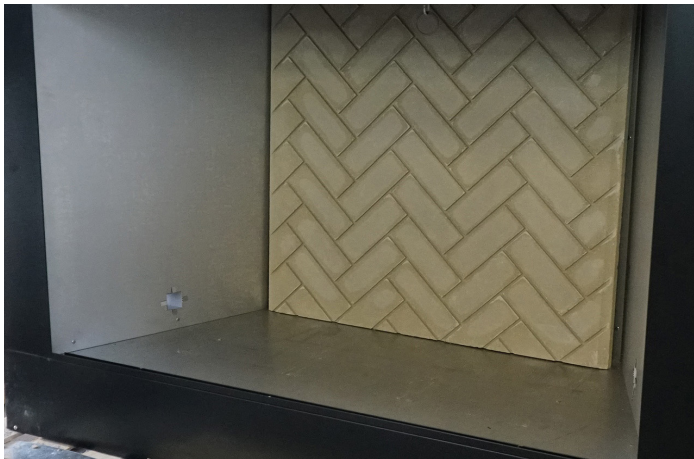
Install Back Refractory Figure 47
