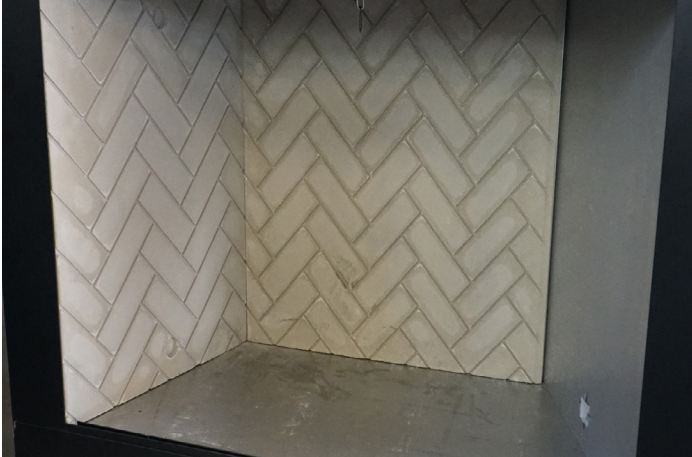
Install Left Side Refractory Brick Liner Figure 50
