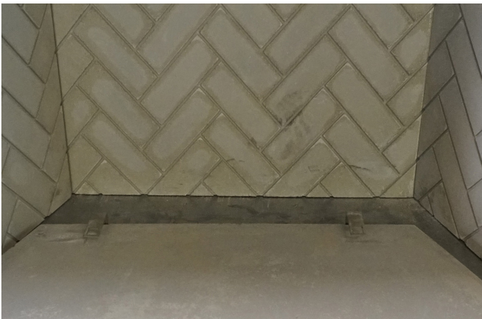
Install Hearth Refractory With Grate Retainers Figure 51
