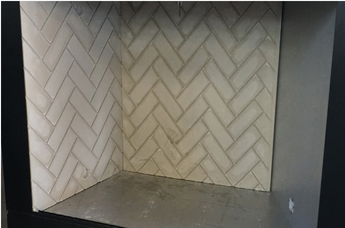
Install Left Side Refractory Brick Liner Figure 50
