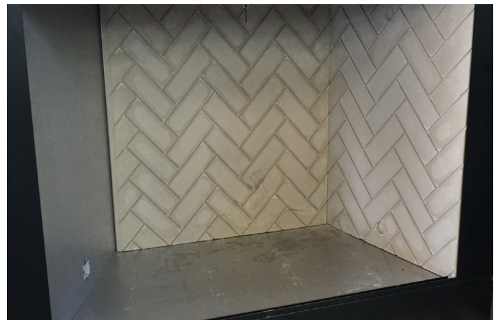
Install Right Side Refractory Brick Liner Figure 49
